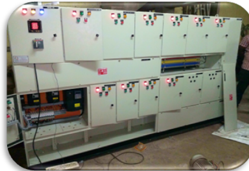
JAYA TV- VFD WITH AUTOMATION PANEL
