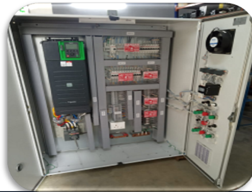
JAYA TV- VFD WITH AUTOMATION PANEL
